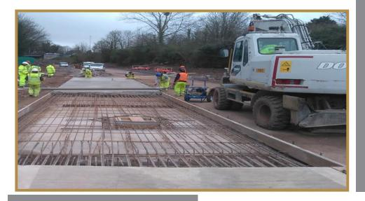
**Scope:** Installation of 6500 m2 of CRCP (Continuously Reinforced Concrete Pavement) and Installation of 64 No. Ground Beam Anchors
