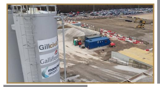
**Scope:** Installation of 7700m2 of 730mm thick type of FH dry lean concrete including 2 no. AGL duct crossing.
